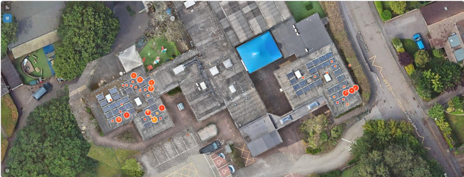
High-resolution visual model with inspection issues mapped directly to the building asset.
